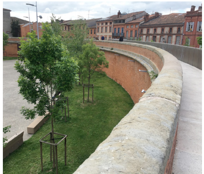
Flood Control structure with pedestrian walkway above in Toulouse.
